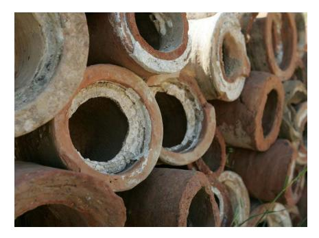
Roman water pipes. They used Terra Cotta pipes, which were easy to create, not toxic like lead pipes and less expensive than stone. Stone blocks with holes bored into them were used for corners and junctions. Site of ancient Ephesus, Turkey.
