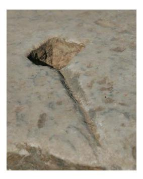
A junction between two sections of a marble column. The sections were joined by short pieces of iron and molten lead was poured down the channels to lock the iron in place. This method of construction was extremely vulnerable to earthquakes, which destroyed most ancient cities in this region. Ancient Ephesus, Turkey.
