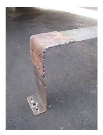
Repaired and reinforced bracket.
