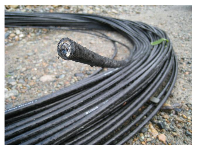
The coil of new optical fiber cable used to patch the cable broken by the flood.
