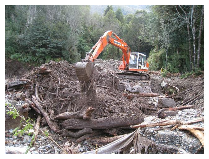
The hoe building the temporary bypass road. Note the size of the debris and boulders.
