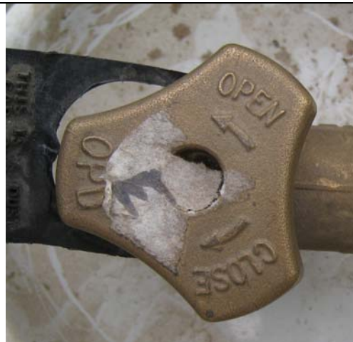
OPD fill valve identified with OPD initials and 3 pronged handle.
